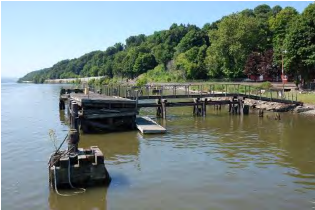
The southern pier at Milton Landing. Image courtesy of Matt Kierstead.
