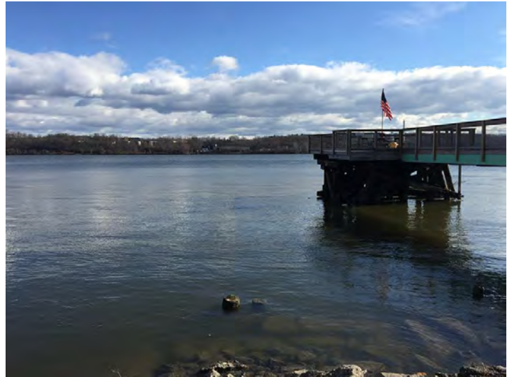
Northern pier at Milton Landing Park in Marlborough provides public access to the Hudson River.
