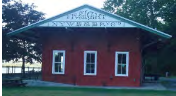
Milton Railroad Station, Milton Landing.
